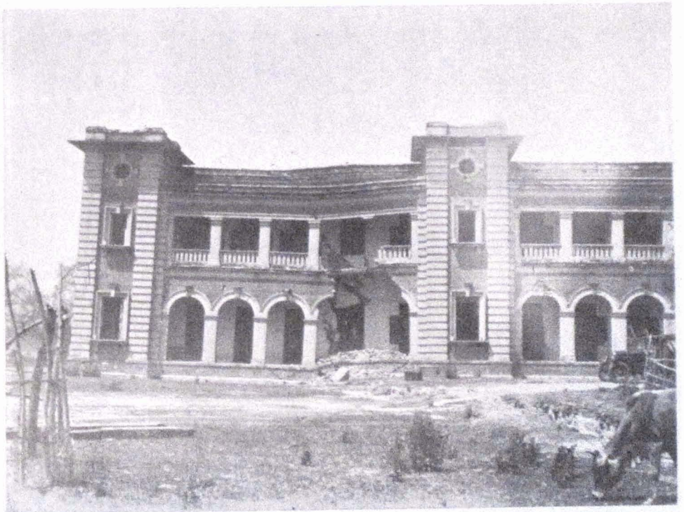
FIG. 2. SLUMPING OF HOUSE, PURNEA.
