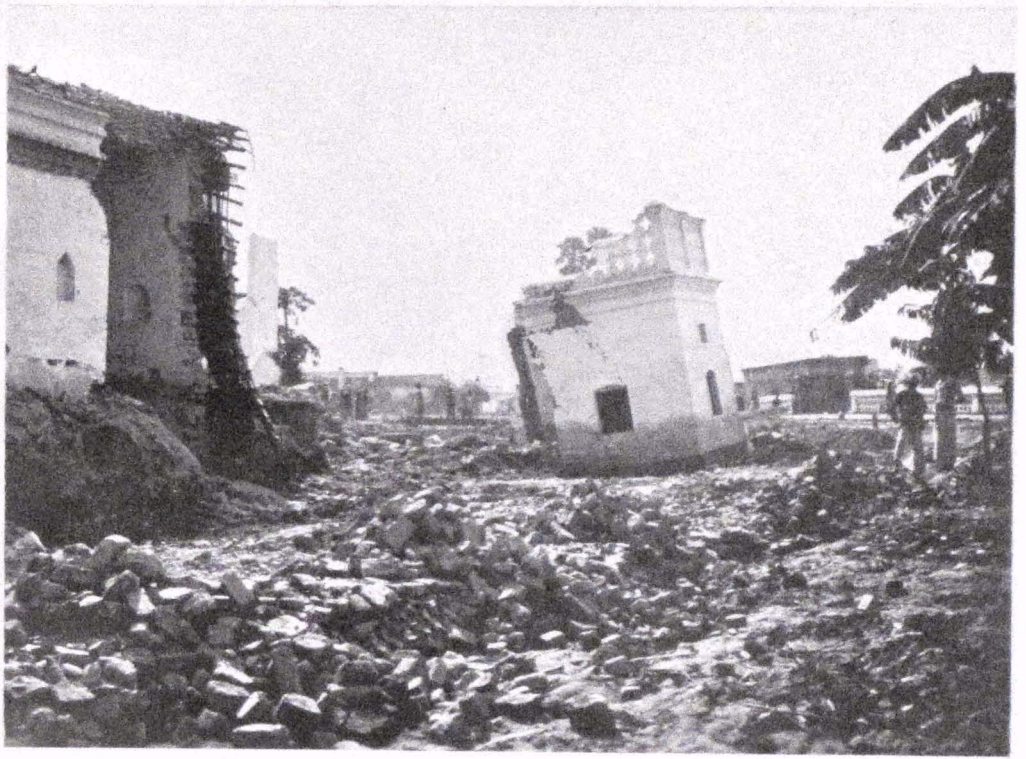
FIG. 1. TILTING OF HOUSES ON FAULT-PLANE IN ALLUVIUM, MOTIHARI.
