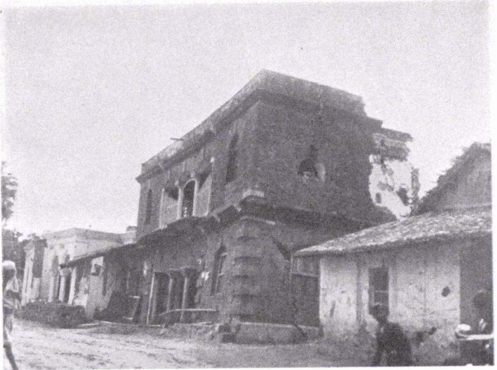
FIG. 1. SLUMPING OF HOUSES, SITAMARHI.
